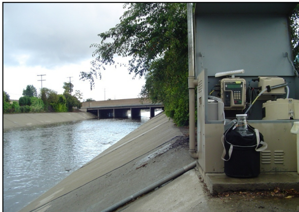
Storm Water Runoff at the Los Cerritos Channel Monitoring Station
