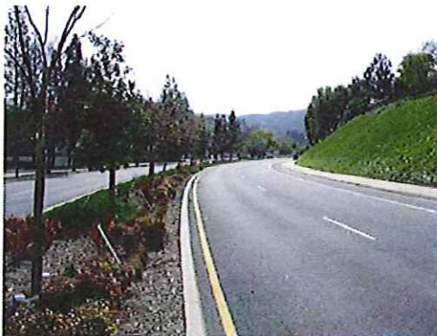
Figure 2: After Photo showing bio-swale eliminating runoff and providing pollutant mitigation via infiltration.
