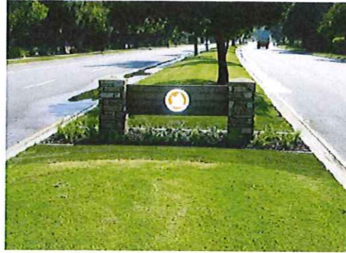
Figure 1: Before Photo with concave design and no infiltration.
