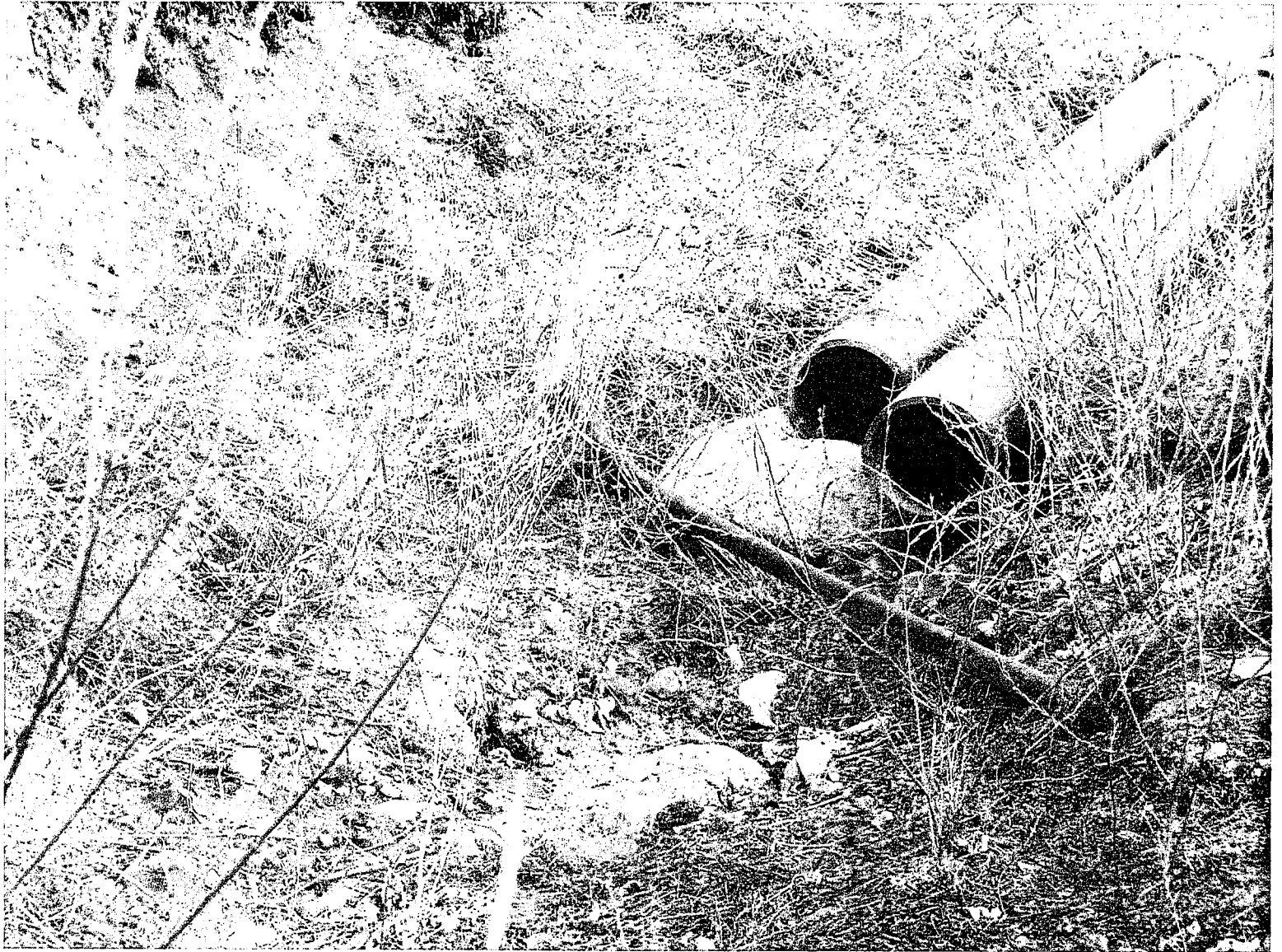
Photo showing unearthed water line leading to neighbor's house from meter at curb on Pinyon.
