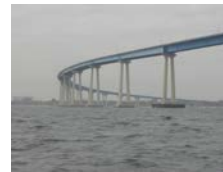
San Diego Bay bridge
