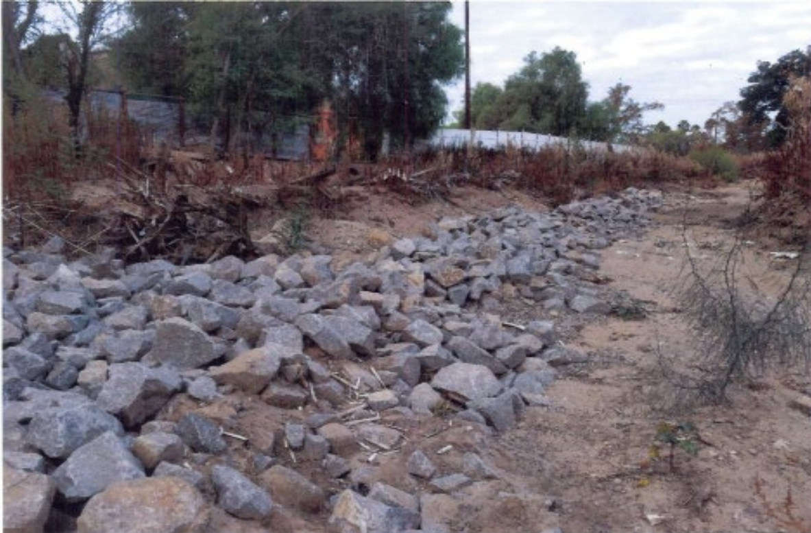
PHOTO 2: Rip rap protection installed in Los Coches Creek channel.
