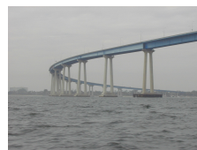
San Diego Bay bridge
