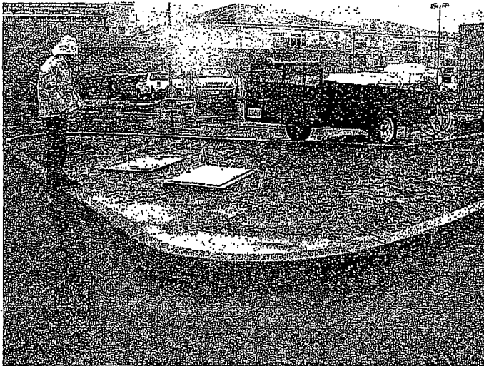
164. Medians in the school parking lot did not have any sediment controls.
