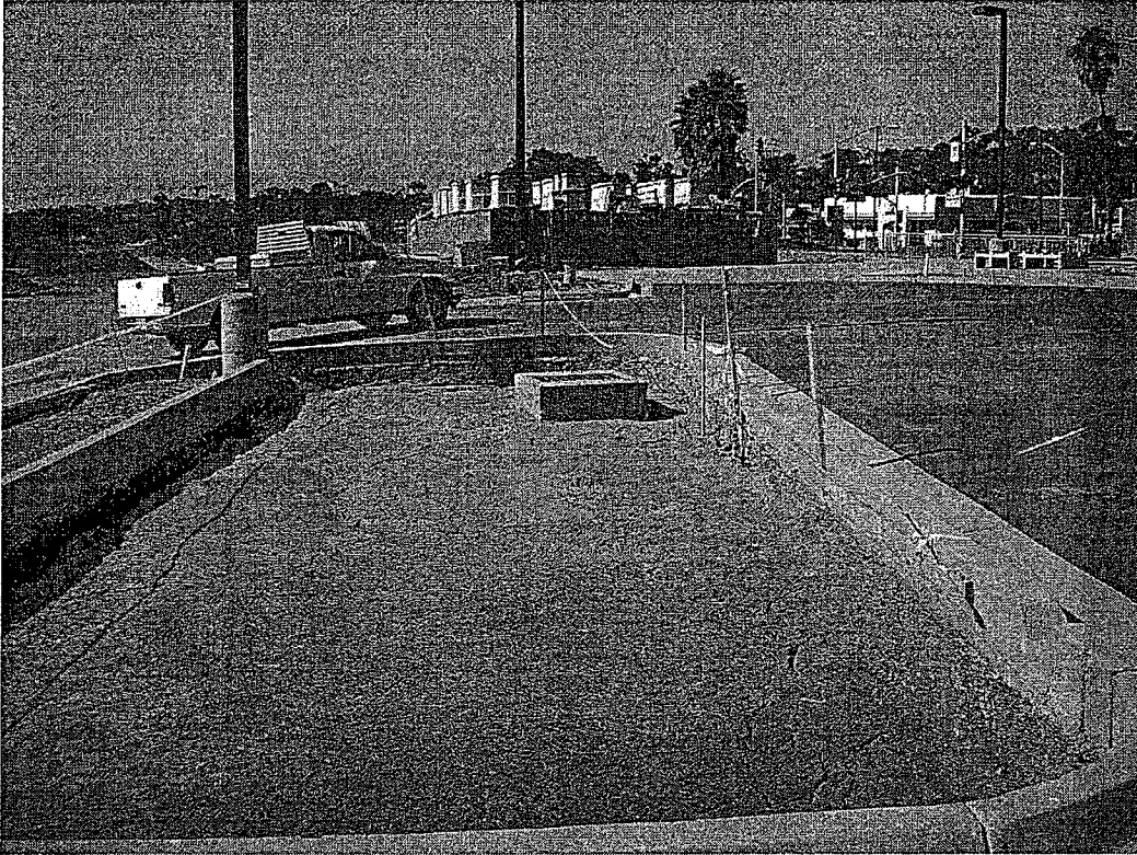
Backfilled with specified soil mix.
