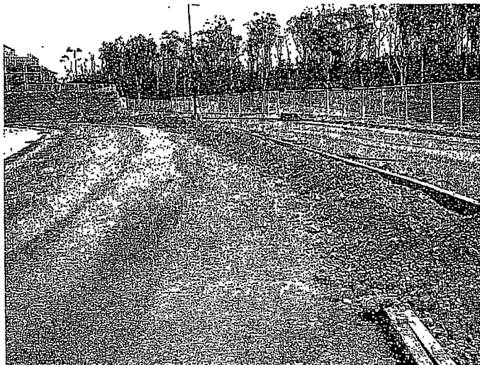
193. Dirt stockpiled on the street with no controls to minimize contact with runoff.
