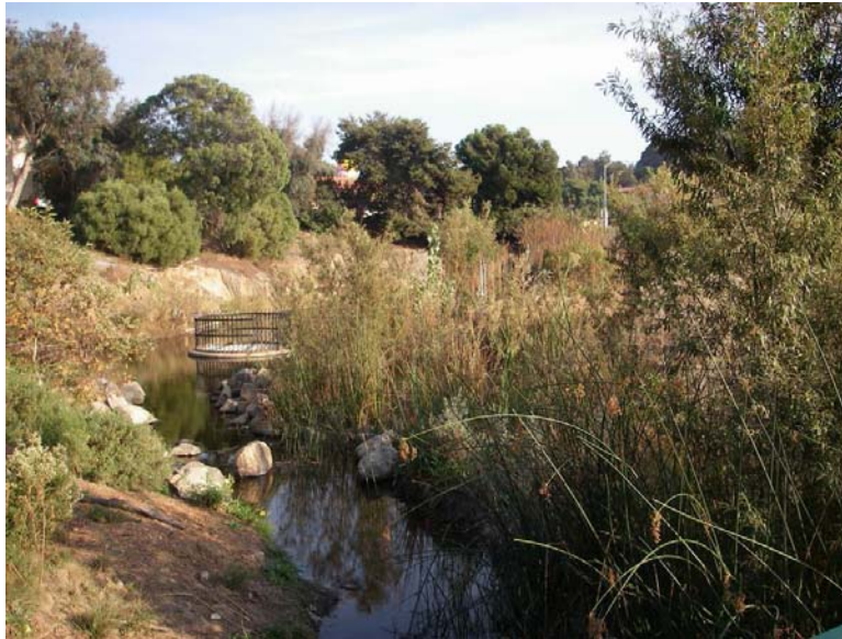
Figure 10. Manufactured Wetlands at Cottonwood Creek Park, Encinitas Blvd., Carlsbad Watershed.
