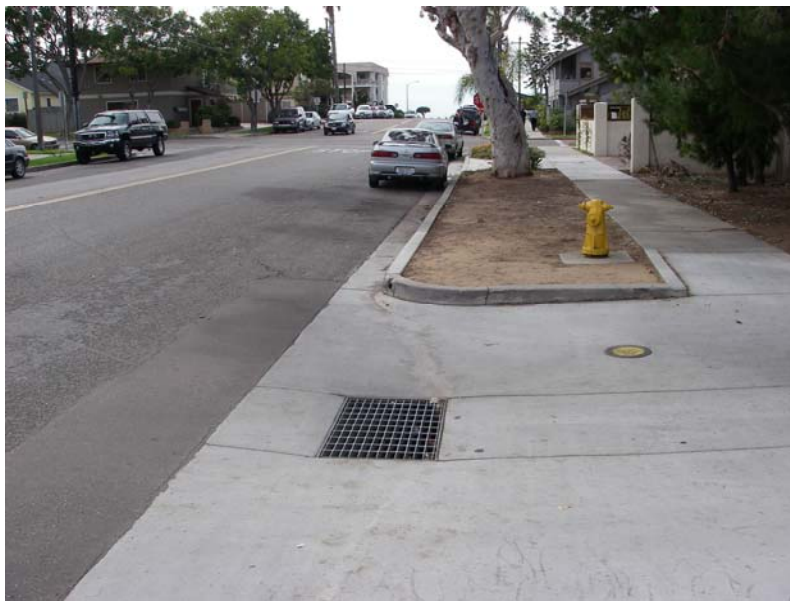
Figure 6. Clean Storm Drain in Residential Area, D Street, Carlsbad Watershed
