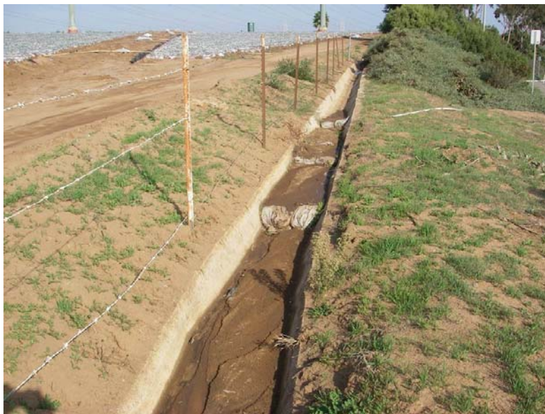
Figure 5. Use of Sandbags near Strawberry Fields, Cannon Rd. near Interstate 5, Carlsbad Watershed.
