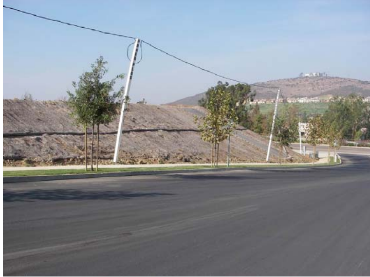
Figure 3. Use of Netting and Fiber Rolls at San Elijo Hills Construction Site, Northstar Way, Carlsbad Watershed.
