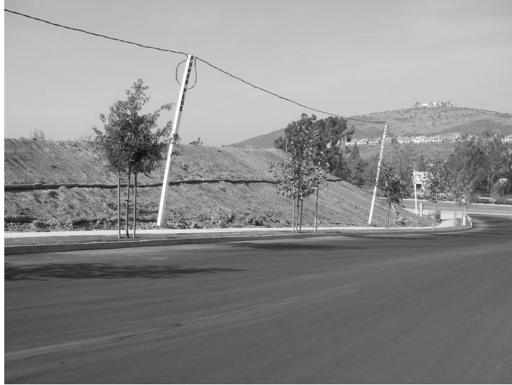
Figure R-3. Use of Netting and Fiber Rolls at San Elijo Hills Construction Site, Northstar Way, Carlsbad Watershed.
