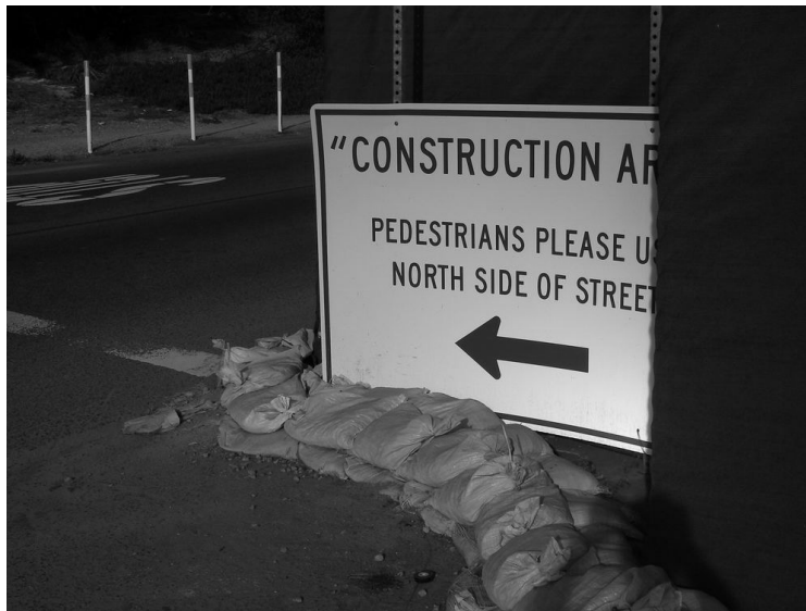
Figure R- 4. Use of Sandbags upstream of Moonlight State Beach, Encinitas Blvd., Carlsbad Watershed.
