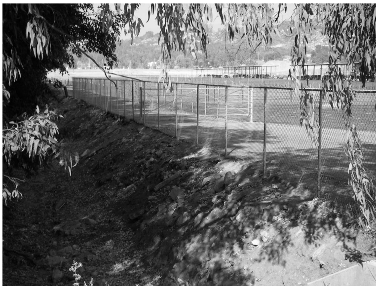
Figure R-1. Animal Exclusion Device at Konyn Dairy, Valley Center Road, San Dieguito Watershed.
