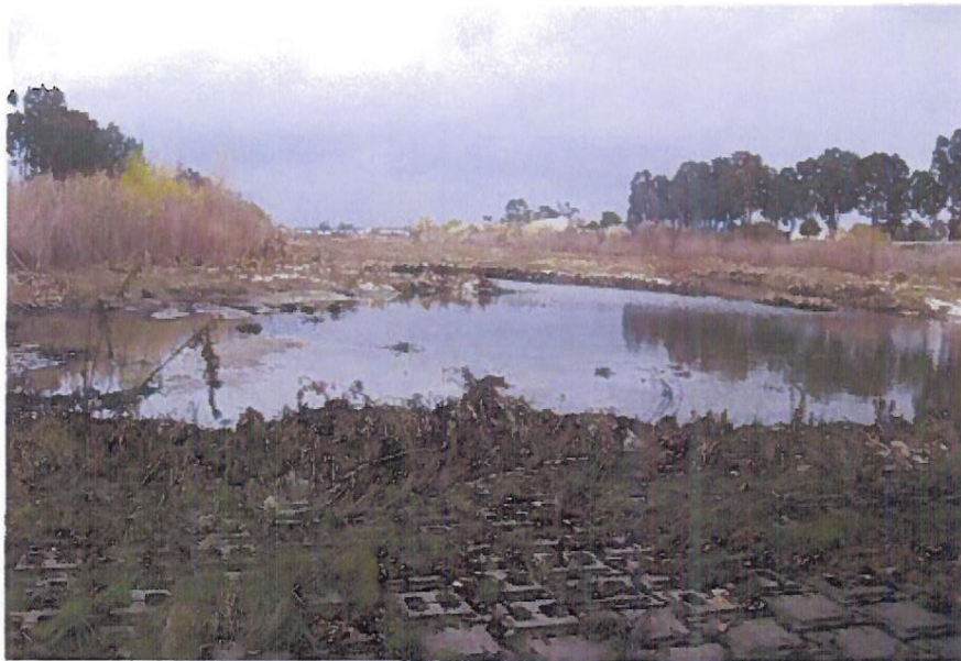
Photo 8. Standing under the Rancho California bridge crossing looking upstream at Murrieta Creek.
