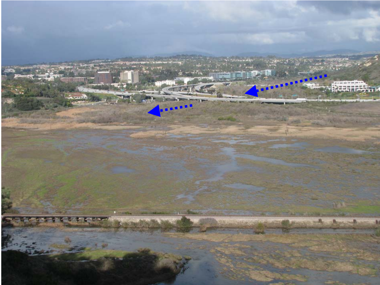
Figure 7. Photograph of Carmel Creek entering Los Peñasquitos Lagoon on January 3, 2011, shortly after a rain event. The creek flows along the dashed arrow, along SR 56 and beneath the I-5 freeway.
