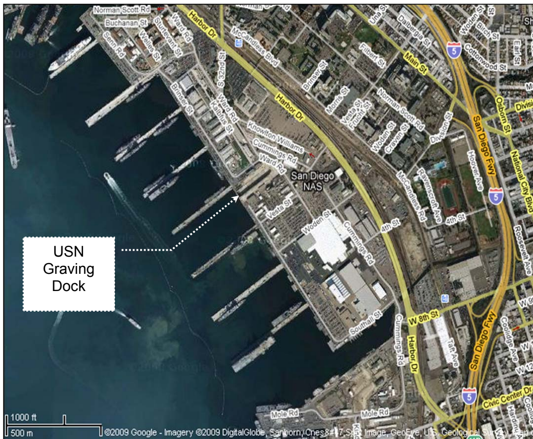
Figure B-9. USN Graving Dock at NBSD
