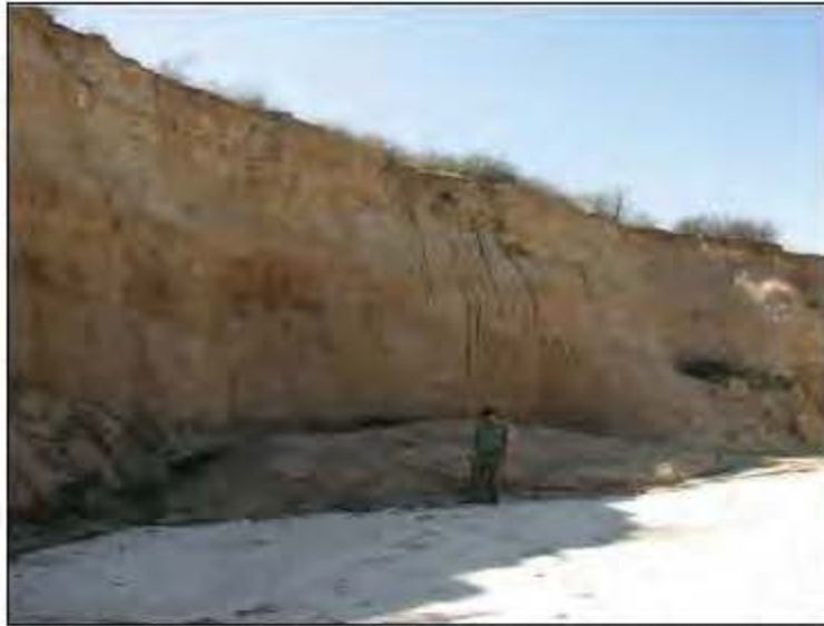
Typical stream erosion in a southern California stream (granular, non-cohesive) (Photo courtesy of Eric Stein, SCCWRP)
