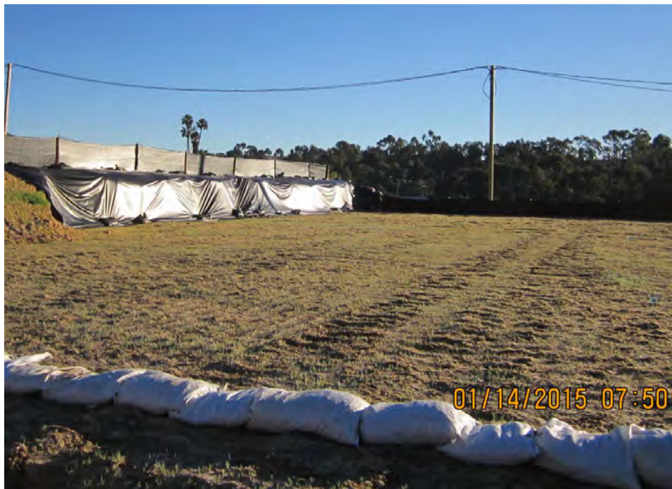
Photo 6 Sidewall protected with plastic sheeting.
