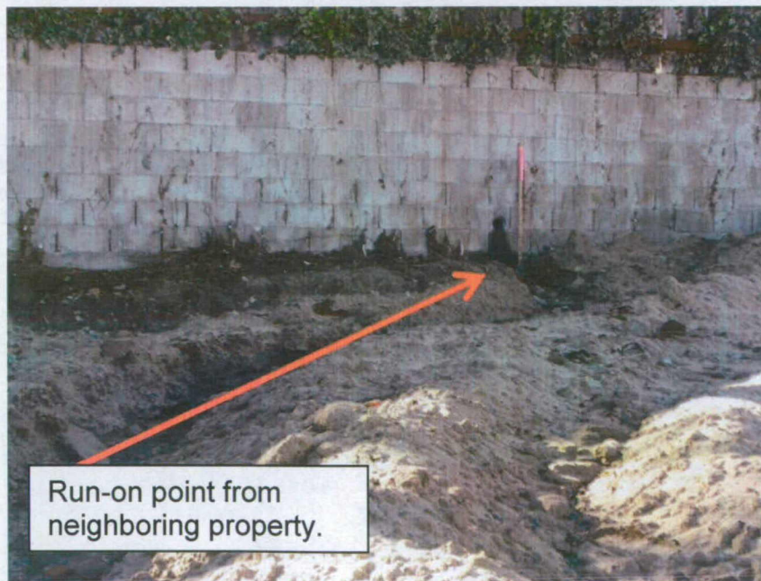
Photo 4: Lack of run-on protection from slope drain from neighboring residence that discharged to dog park area.
