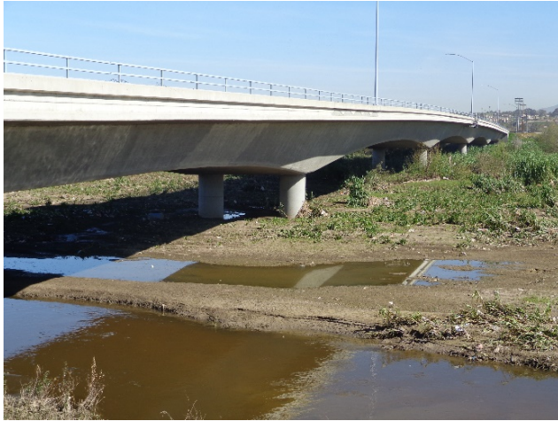
Figure 5 Tijuana River at Dairy Mart Bridge
