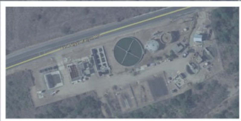
USMC Sewage Treatment Plant 9
