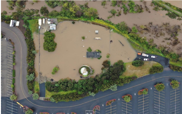
Figure 3. Buena Vista Lift Station April 10, 2020.
