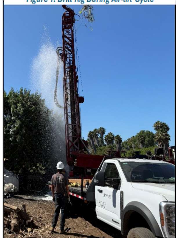
Figure 1: Drill Rig During Air-lift Cycle
