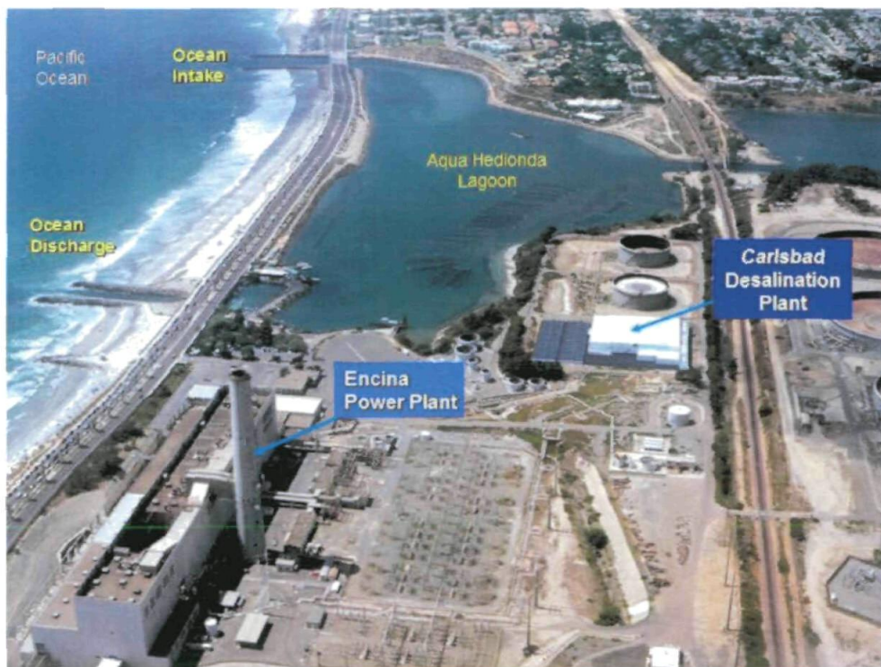
Figure 1 – Carlsbad Seawater Desalination Project
