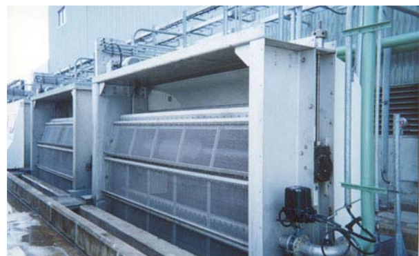
Figure 6. An example of a traveling screen (company name omitted to prevent bias; image obtained from freeshare website)
