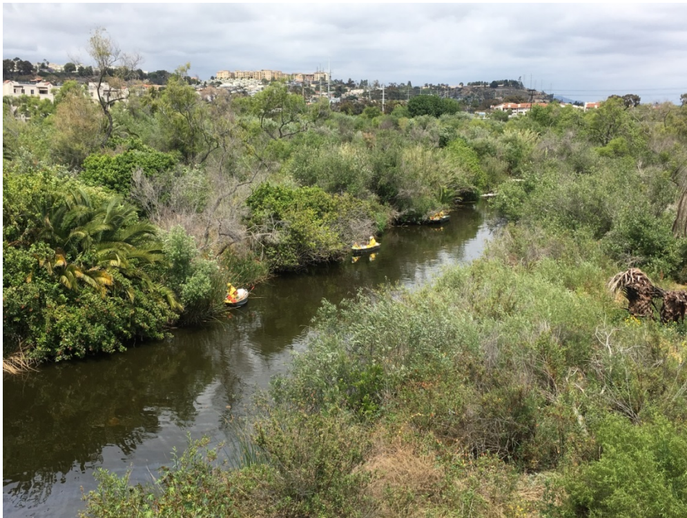
Figure 3: Emergency response team removing and cleaning diesel impacted vegetation along the San Diego River.
