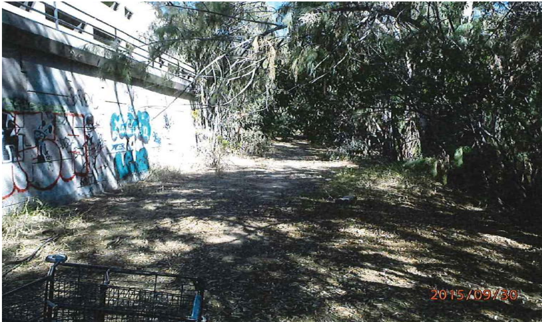
Pre-project photo looking upstream- Dense vegetation with scattered trash from homeless encampments.
