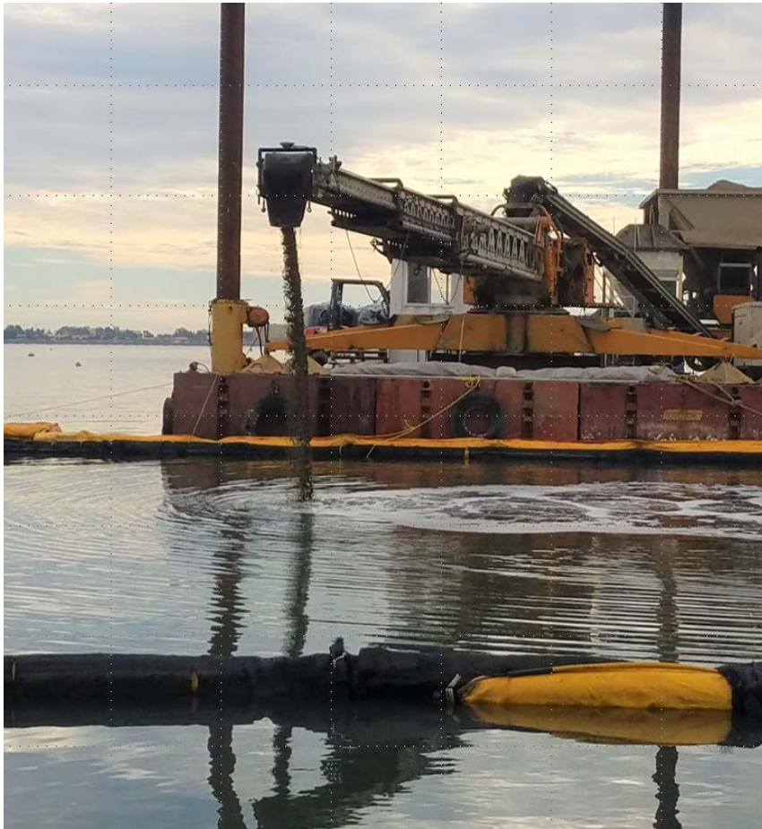
Placement of Thin Layer Cover (EMNR)
