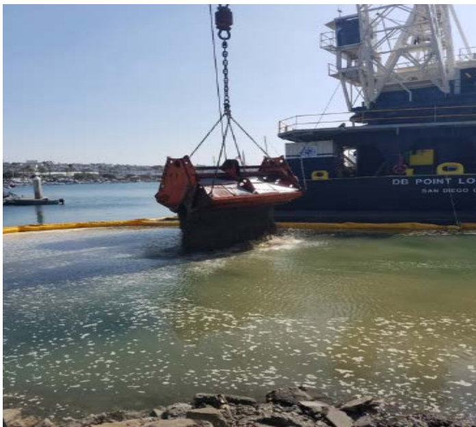
Clean Sand Backfill Placement in the dredged area
