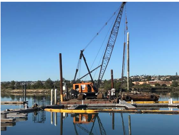
Figure 2: MCRD Boat Dock following final inspection (Photo provided by Department of Navy)
