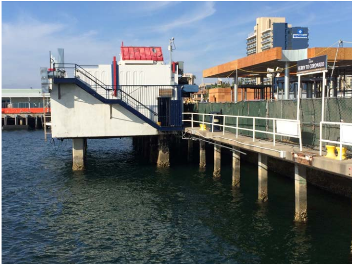
View to the north.
