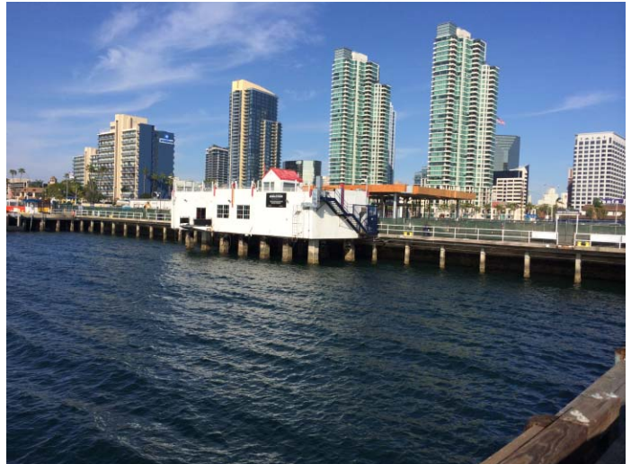
View from the southwest.
