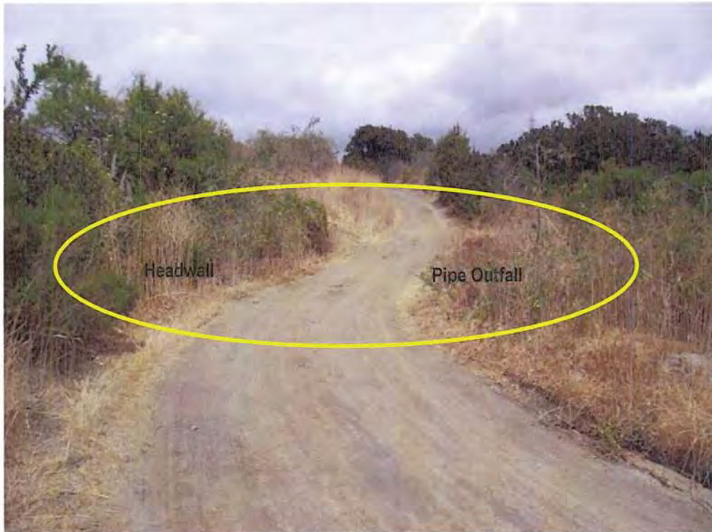
Figure 1. North-facing overview of road repair location.
