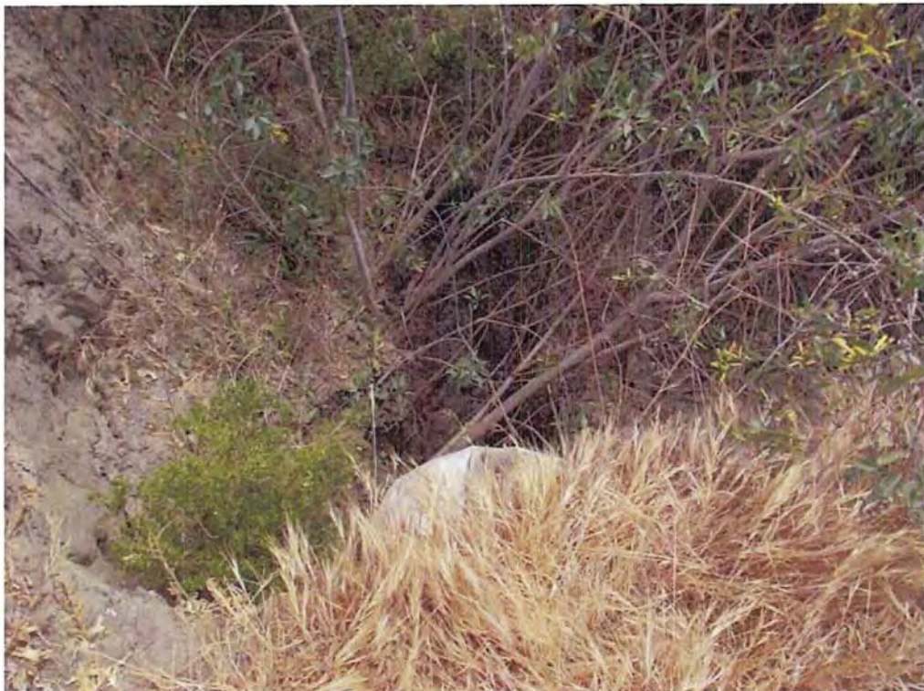
Figure 2. East-facing view of drainage channel at outfall pipes.
