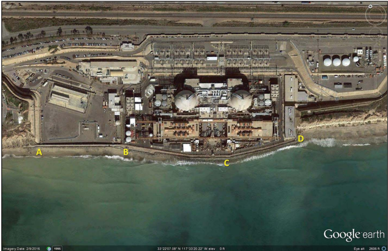
Figure 2. The public beach walkway is situated along the west (seaward) perimeter of San Onofre Nuclear Generating Station, sections of which are denoted by letters A through D. The North Industrial Area walkway comprises sections A (north entrance of walkway) to B. Section B marks the beginning of the Units 2/3 walkway and ends at D. The length between sections C to D is the area of highest need of riprap repair.
