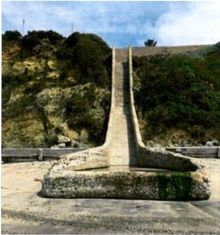
Photo 1. Drainage chute at MP 244.4 during summer months.
