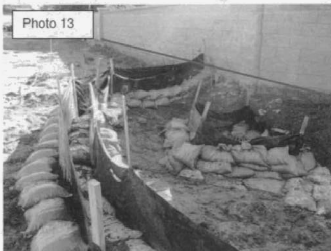
Photo 13 and 14 show new gravel bags (green bags) were placed after the rain event and prior to the inspection. The outer most silt fence was also placed after the rain event and prior to the inspection. The middle silt fence has sediment all over it indicating it was in place before the rain event. The outer most silt fence and stakes were clean. This area was inundated with sediment laden water as indicated by the sediment line on the brick wall (red line). The elevation of the red line is well above the storm drain inlet indicating a discharge of site sediment to the storm drain.
