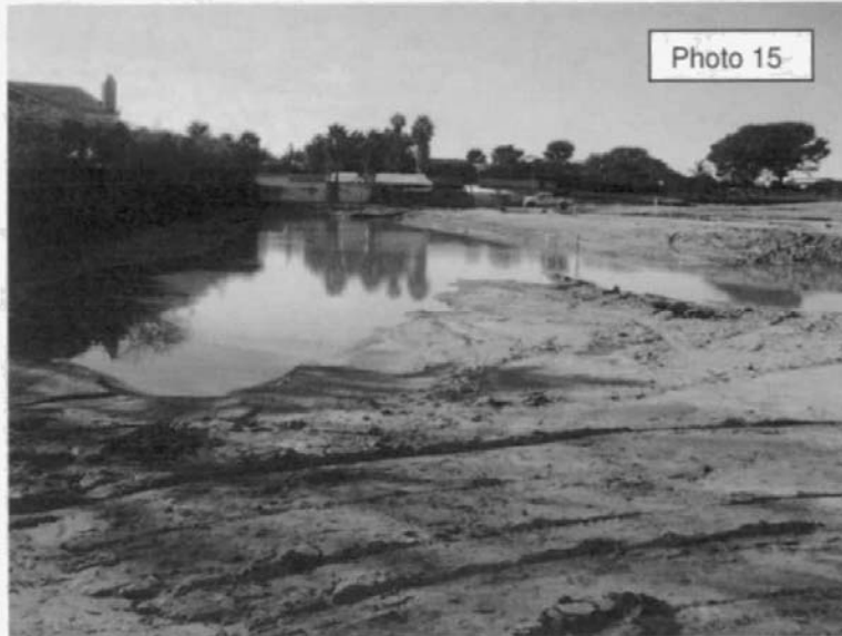
Photo 15 shows reported location where a sediment basin will be constructed.
