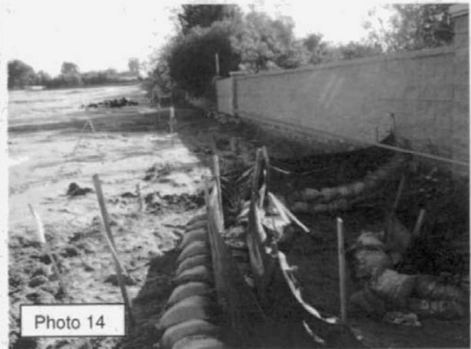
Photo 13 and 14 show new gravel bags (green bags) were placed after the rain event and prior to the inspection. The outer most silt fence was also placed after the rain event and prior to the inspection. The middle silt fence has sediment all over it indicating it was in place before the rain event. The outer most silt fence and stakes were clean. This area was inundated with sediment laden water as indicated by the sediment line on the brick wall (red line). The elevation of the red line is well above the storm drain inlet indicating a discharge of site sediment to the storm drain.
