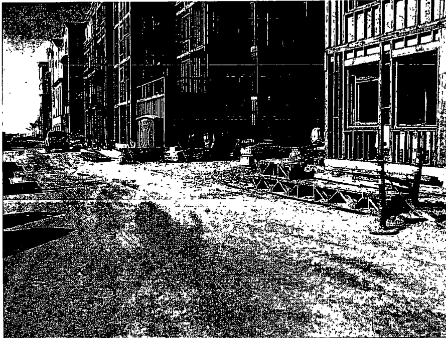
Figure 1. South side of active construction site
