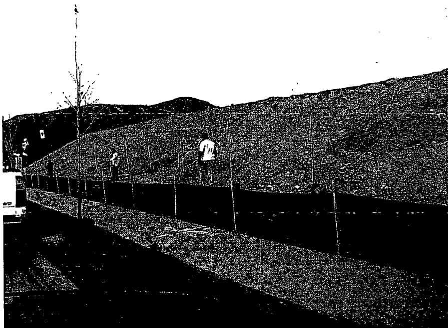
Figure 12. Slope on west side of property
