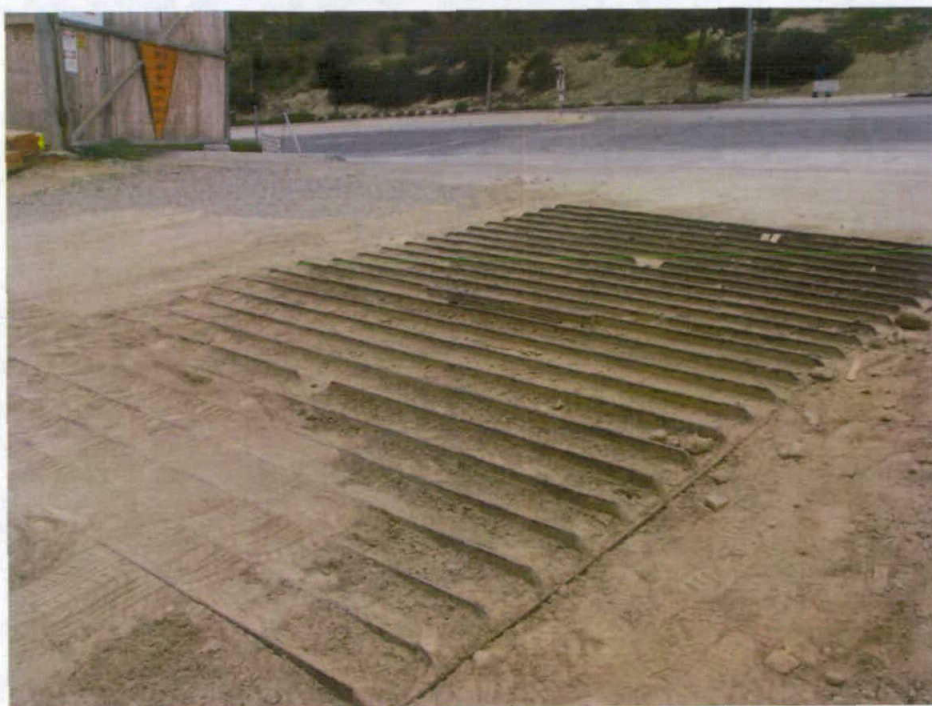
Figure 15. Shaker plates north entrance
