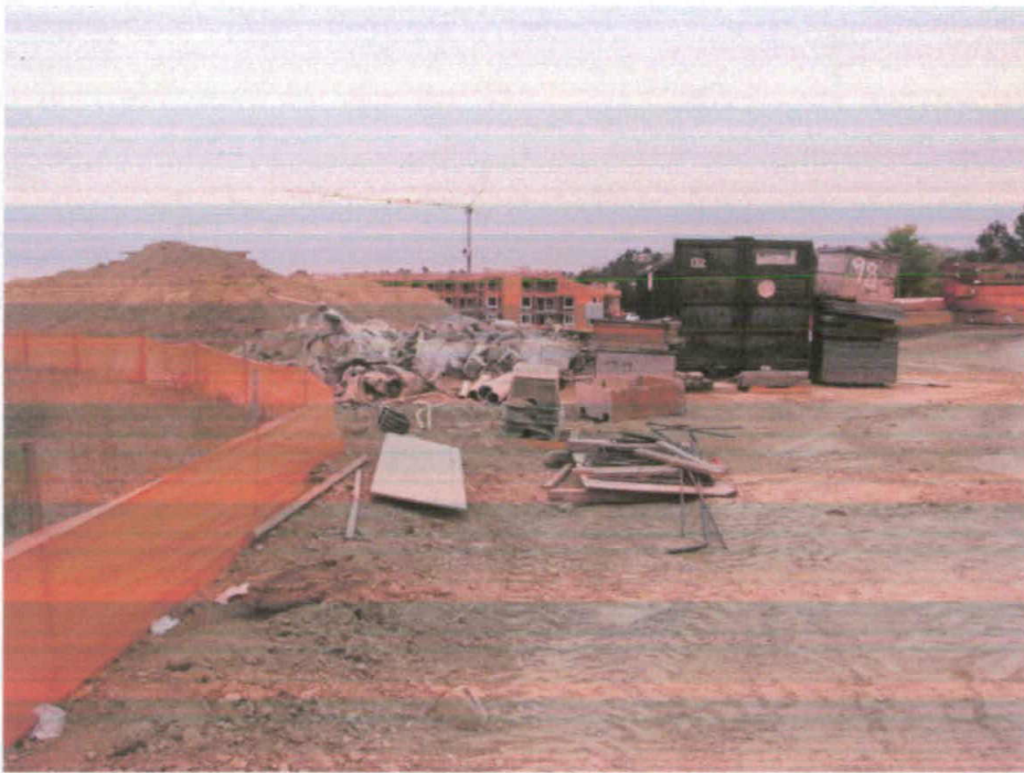
Figure 5. Site interior; construction debris
