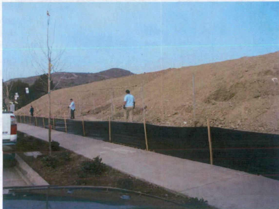
Figure 12. Slope on west side of property
