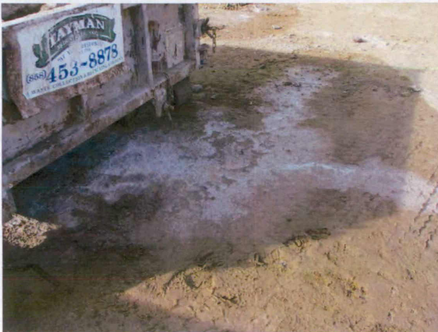
Figure 8. Concrete staining on soil from leaking washouts
