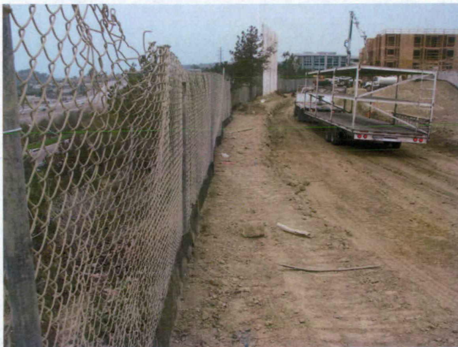
Figure 11. Perimeter west side
