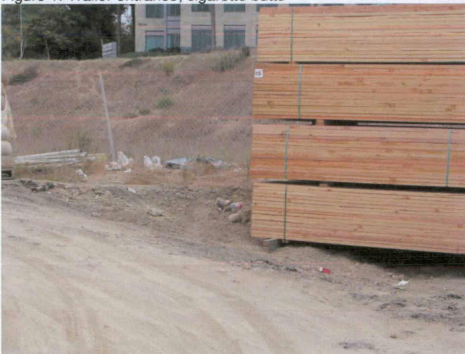
Figure 2. Near south entrance; trash area
