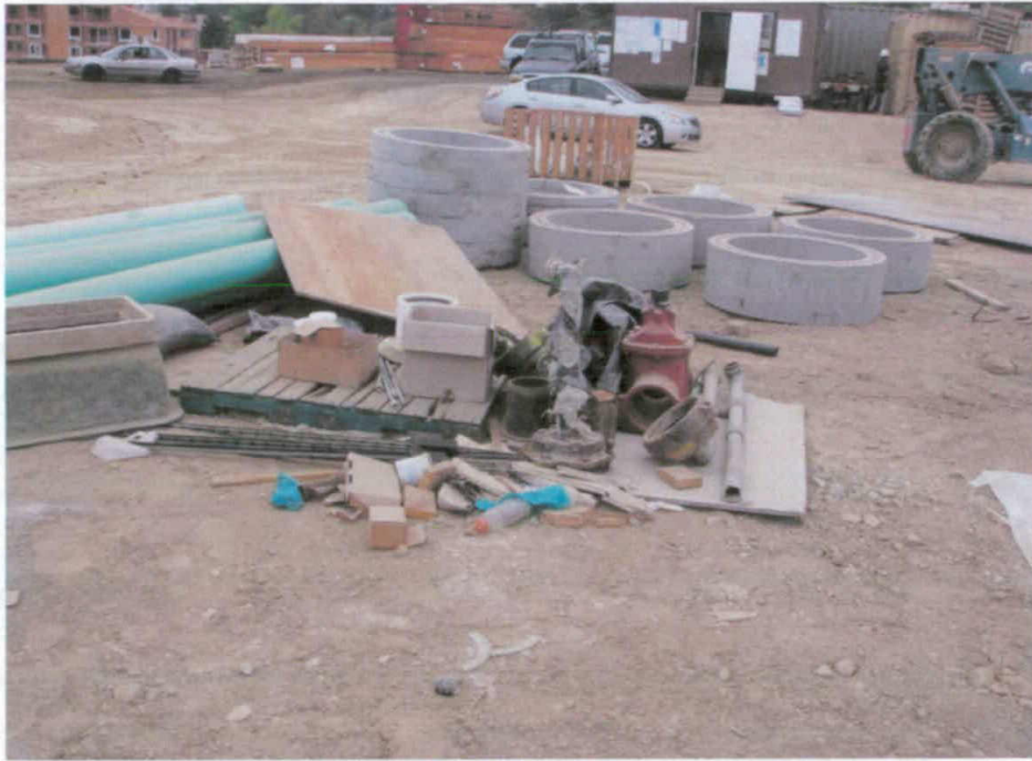
Figure 3. Site interior; construction debris
