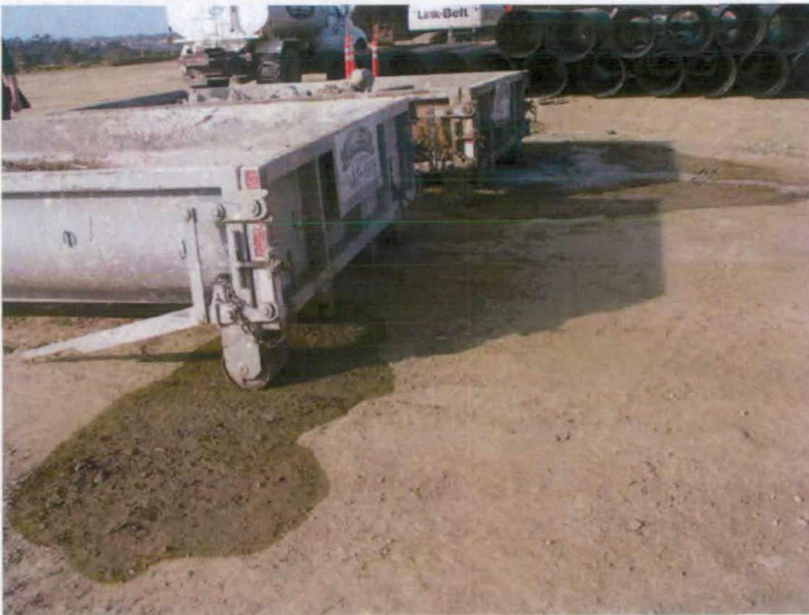
Figure 7. Leaking concrete washouts
