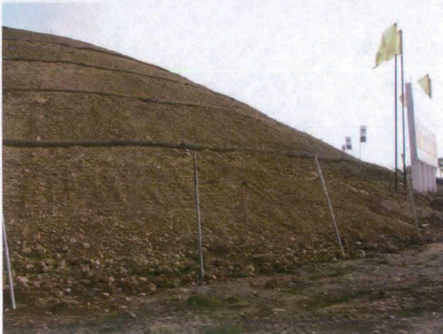
Figure 10. Slope is 2:1 Horizontal: Vertical according to SWPPP
