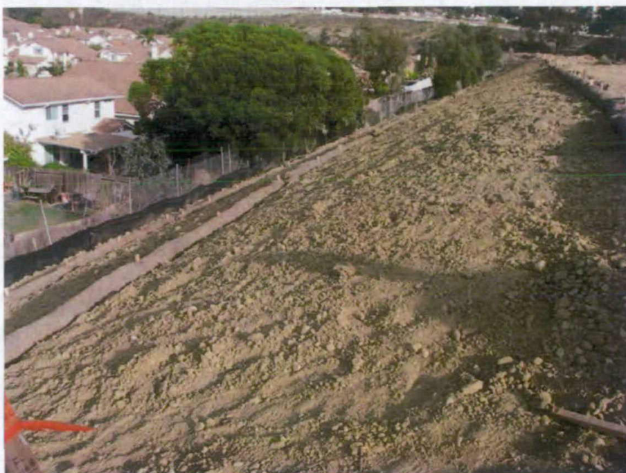
Figure 11. North slope looking easterly
