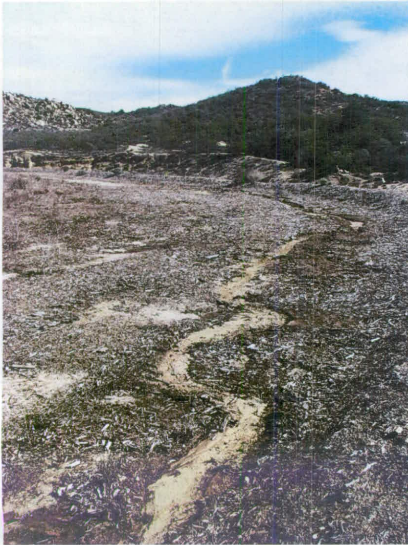
Erosion along the top deck of the landfill. A lack of BMPs and storm water management has caused erosion along the perimeter of the top deck. Photo taken January 14, 2016 during a site inspection.
