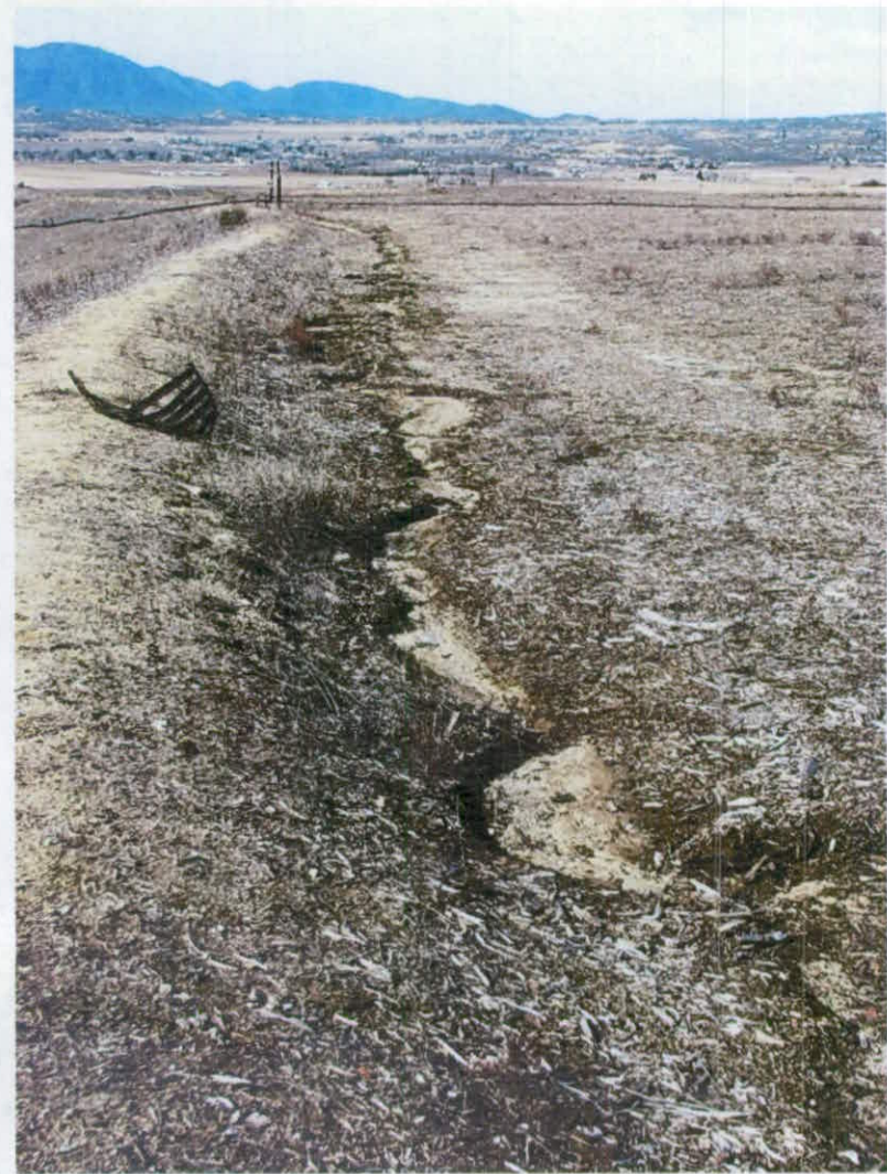
Erosion along the top deck of the landfill. A lack of BMPs and storm water management has caused erosion along the perimeter of the top deck. Photo taken January 14, 2016 during a site inspection.
