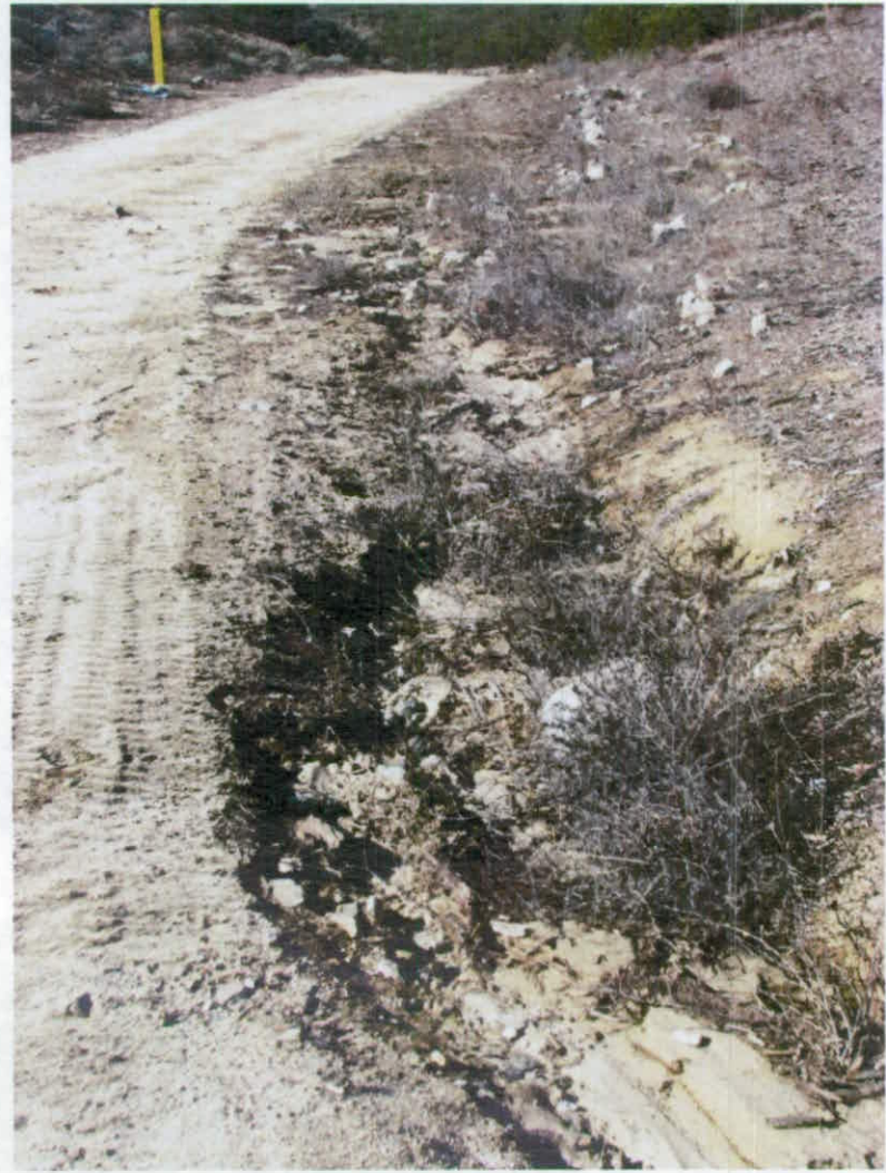
Erosion along the middle bench (left photo) and lower bench (right photo) caused by unmanaged storm water flows. Photo taken January 14, 2016 during a site inspection.
