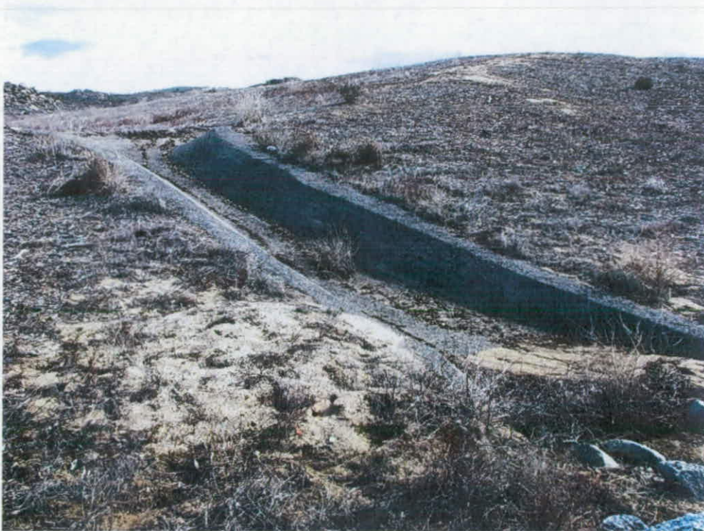
Drainage Swale from the upper deck to the middle bench (top photo) and from the upper deck looking down the entire side slope (lower photo). Drainage swale is full of debris which should be removed prior to the next storm event to promote positive flow and drainage to the desiltation basin. Photo taken January 14, 2016 during a site inspection.
