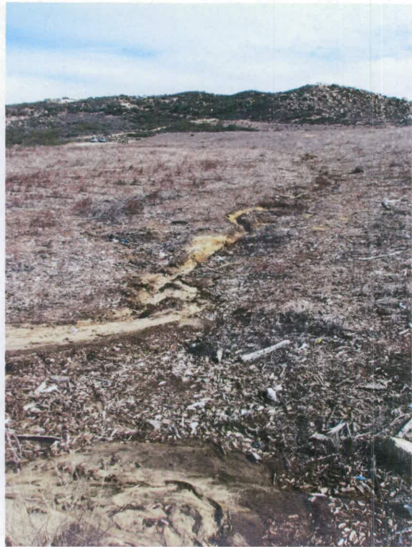
Erosion along the upper deck leading to a drainage swale designed to carry storm water runoff to the desiltation basin at the toe of the landfill. Photo taken January 14, 2016 during a site inspection.
