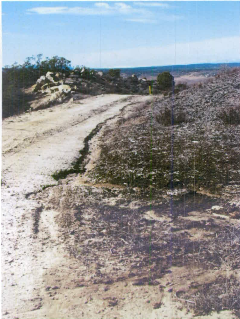
Erosion along the bench/service road caused by unmanaged storm water flows. Photo taken on January 14, 2016 during a site inspection.
