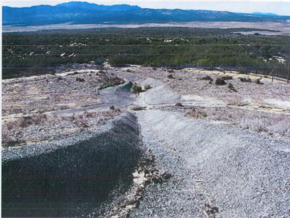
Drainage Swale from the upper deck to the middle bench (top photo) and from the upper deck looking down the entire side slope (lower photo). Drainage swale is full of debris which should be removed prior to the next storm event to promote positive flow and drainage to the desiltation basin. Photo taken January 14, 2016 during a site inspection.
