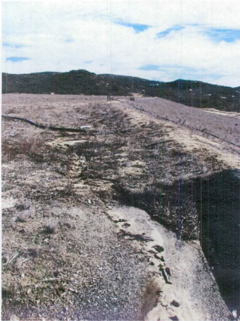
Erosion along the upper deck leading to a drainage swale designed to carry storm water runoff to the desiltation basin at the toe of the landfill. Photo taken January 14, 2016 during a site inspection.
