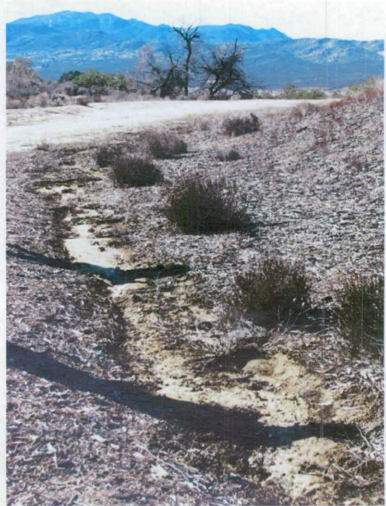
Erosion along the bench/service road caused by unmanaged storm water flows. Photo taken on January 14, 2016 during a site inspection.
