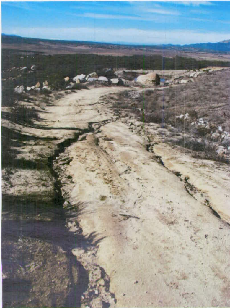
Erosion along lower bench caused by unmanaged storm water flows. Photo taken January 14, 2016 during a site inspection.
