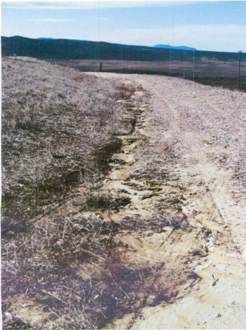
Erosion along the middle bench (left photo) and lower bench (right photo) caused by unmanaged storm water flows. Photo taken January 14, 2016 during a site inspection.
