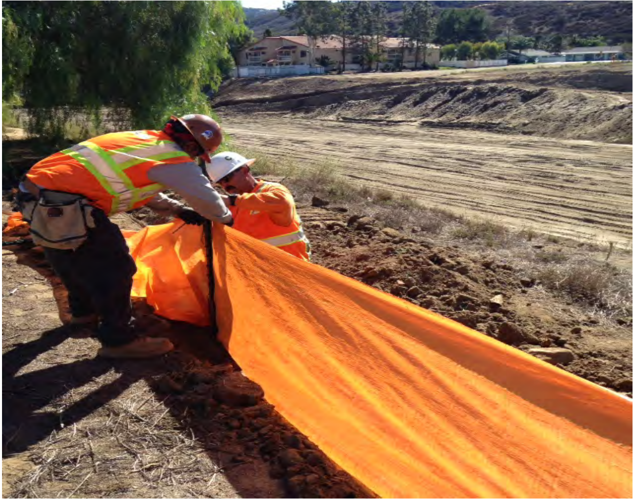
Crews installing additional silt fence along east bank Approx. Sta. 78+00 to 72+00.
