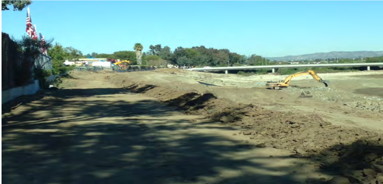
Picture shows riprap being installed as part of the permanent slope protection from Sta. 102+00 to 98+00. The earthen berm on top along the access road is a part of the temp. run-on control.
