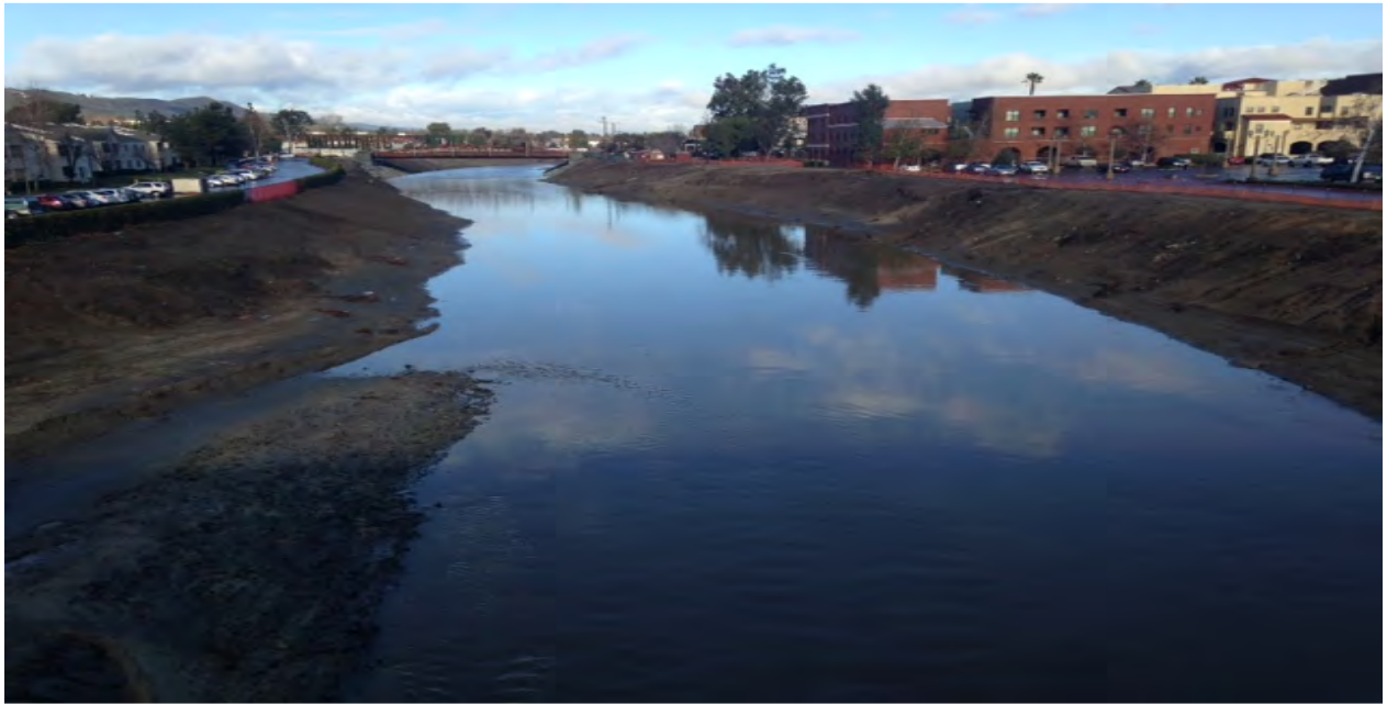
Picture is looking upstream from 1 st St. Bridge on 1/7/16.
