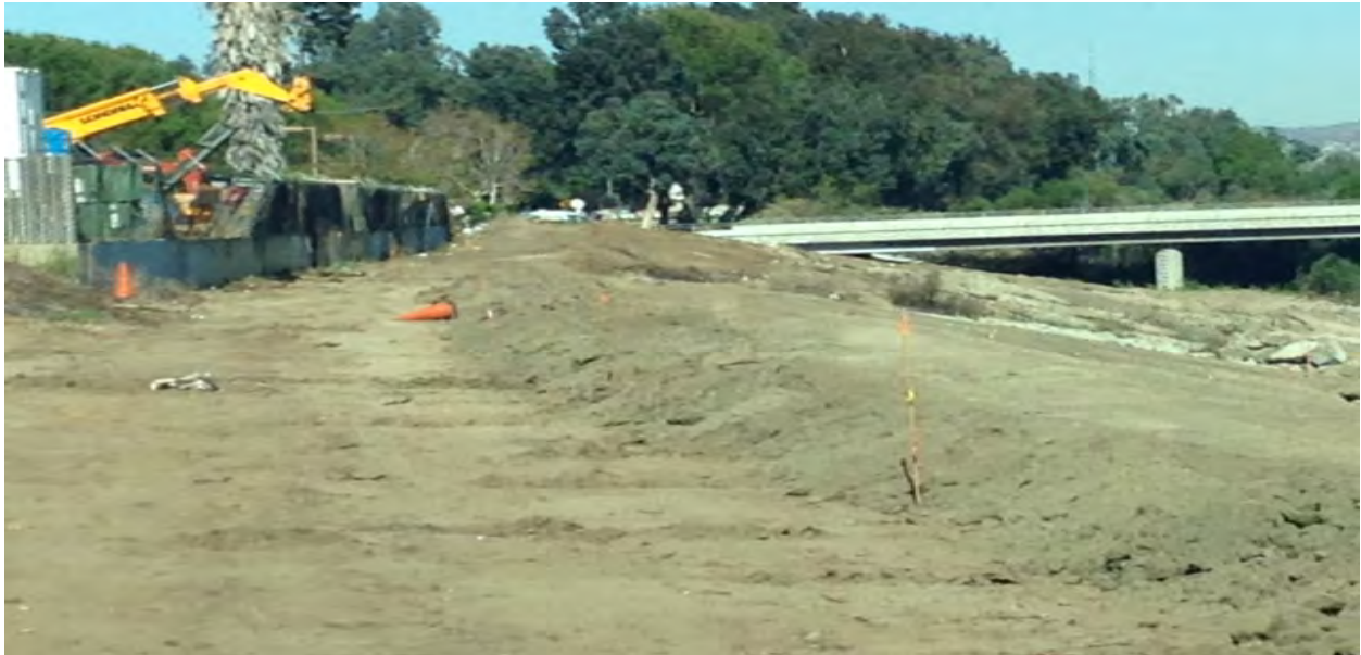
Earthen berms are placed on top of embankments in non-active parts of the creek as part of the run-on protection. North end of the project near Rancho California Rd. This portion of the project from Sta. 107+00 to 102+00 is to be cleared only. OHL has requested US Army Corp to review the current condition and provide contour grading plans as well as any recommended BMPs.
