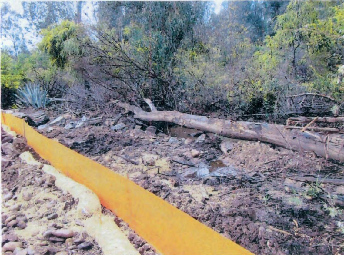
Photo 7 –Construction activities and debris have entered entering waters of the United States and/or State.
