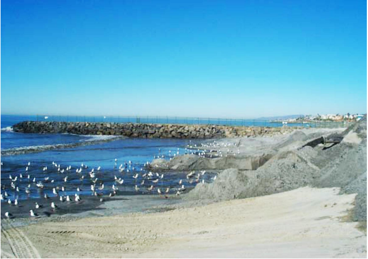
Figure 4: Disposal activities of Agua Hedionda Lagoon dredge sands on South Beach. (photo courtesy of NRG Energy).
