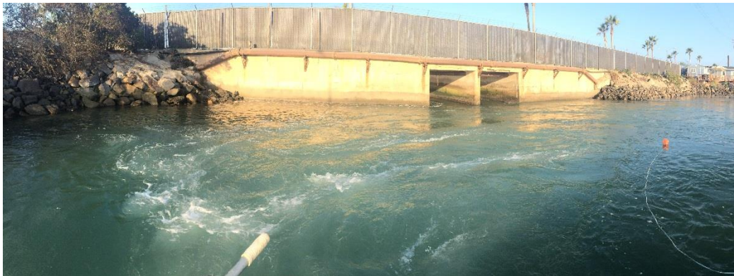
Aeration in the Discharge Pond
