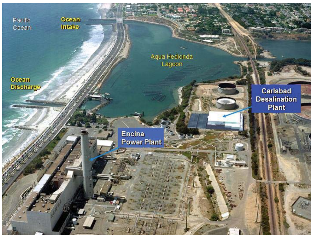
Figure 1 - Carlsbad Seawater Desalination Project
