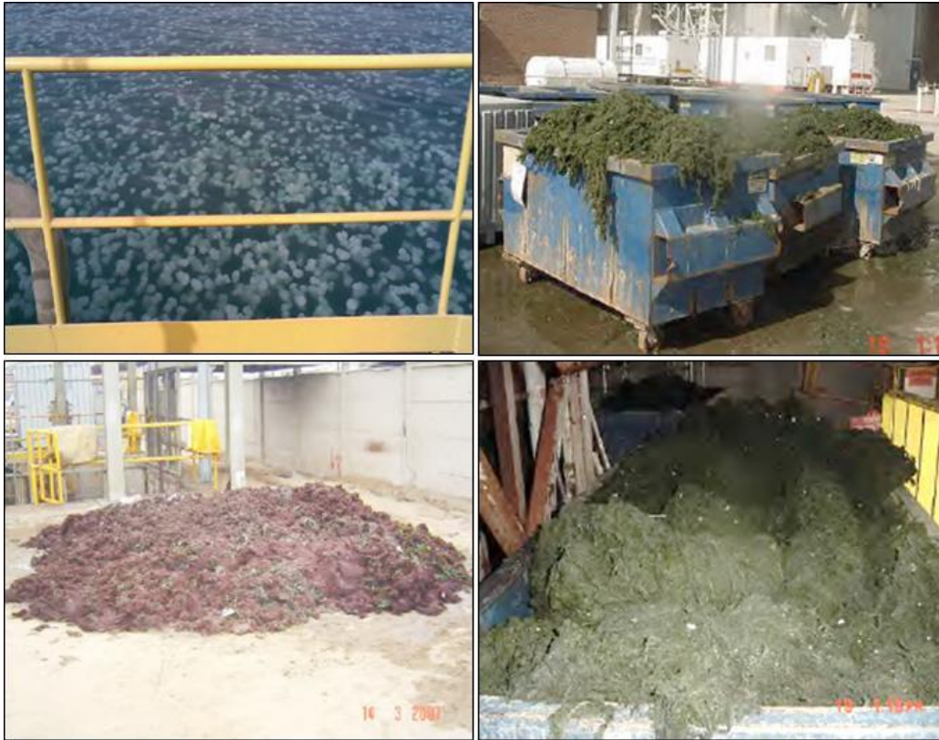
Figure 2. Photographs of seawater intake debris collected by BWT intake screening equipment.
