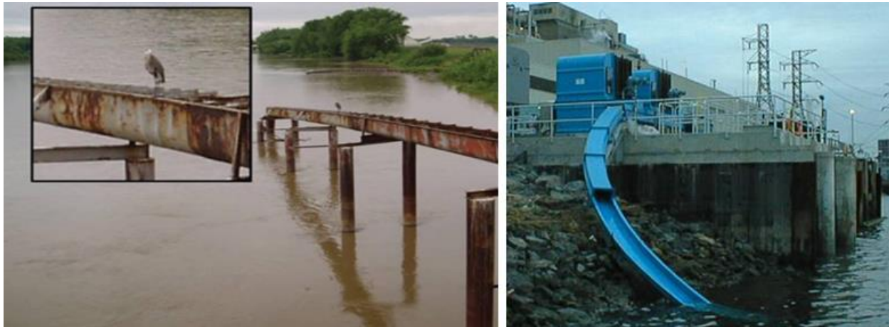
Figure 3. Avian predator perched on fish return system (left) and fish return properly covered to minimize risk of avian predation (right). Note that the image on the right shows the return trough uncovered up to the high water line so that discharge is always free surface regardless of tidal elevation.
