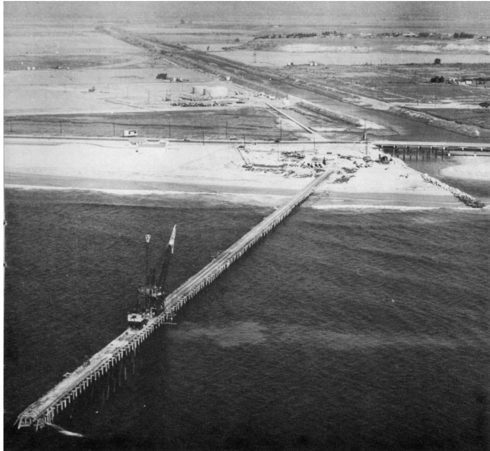
Figure 3.3 Typical trestle construction
