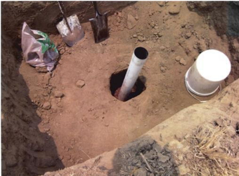
Figure VII.17. Photo of Percolation Test Pit.
