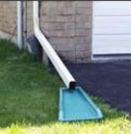
Simple Downspout Dispersion Source: toronto.ca/environment/water.htm
