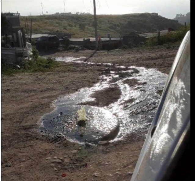
Ongoing raw sewage overflow in residential neighborhood of Tijuana
