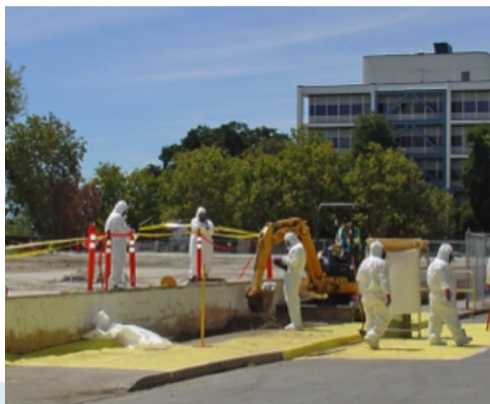
Photo above: Removal of mercury from soil at Lawrence Livermore National Laboratory, a DoE site
