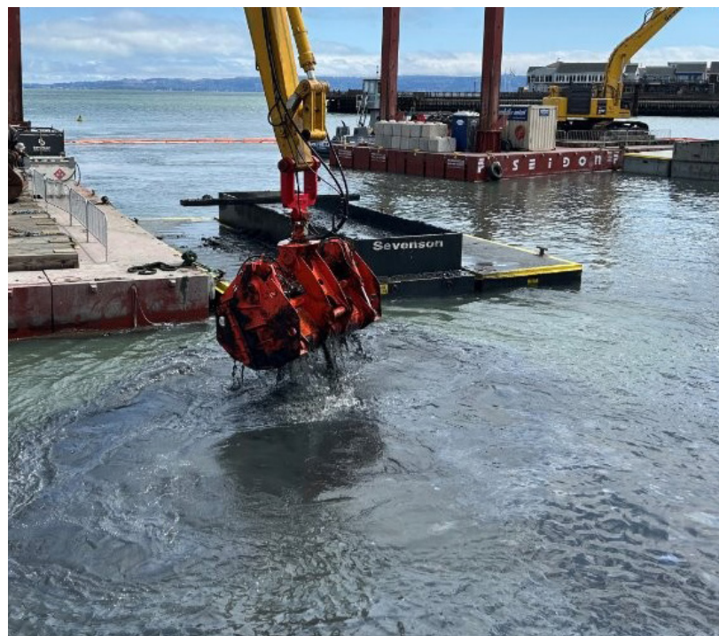
Photo above: Sediment excavation at Pier 39, San Francisco
