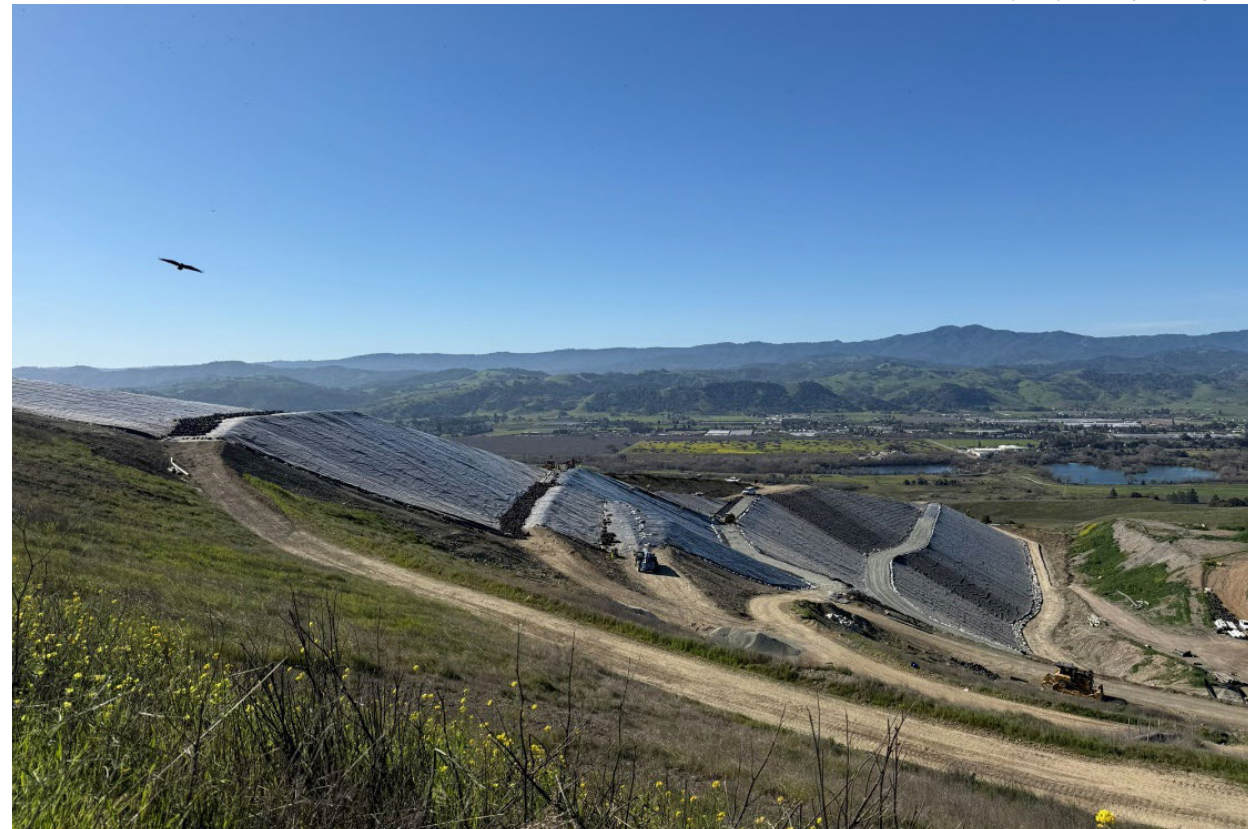
Photo below: Kirby Canyon Landfill, Morgan Hill
