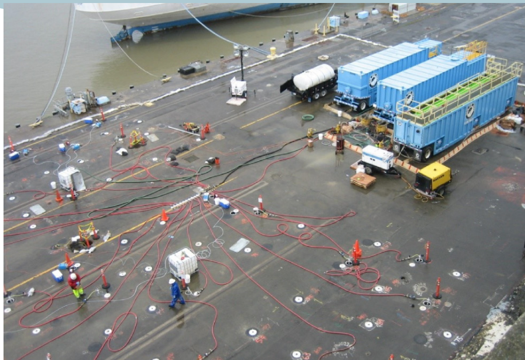
Photo below: Remedial injections at Mare Island
