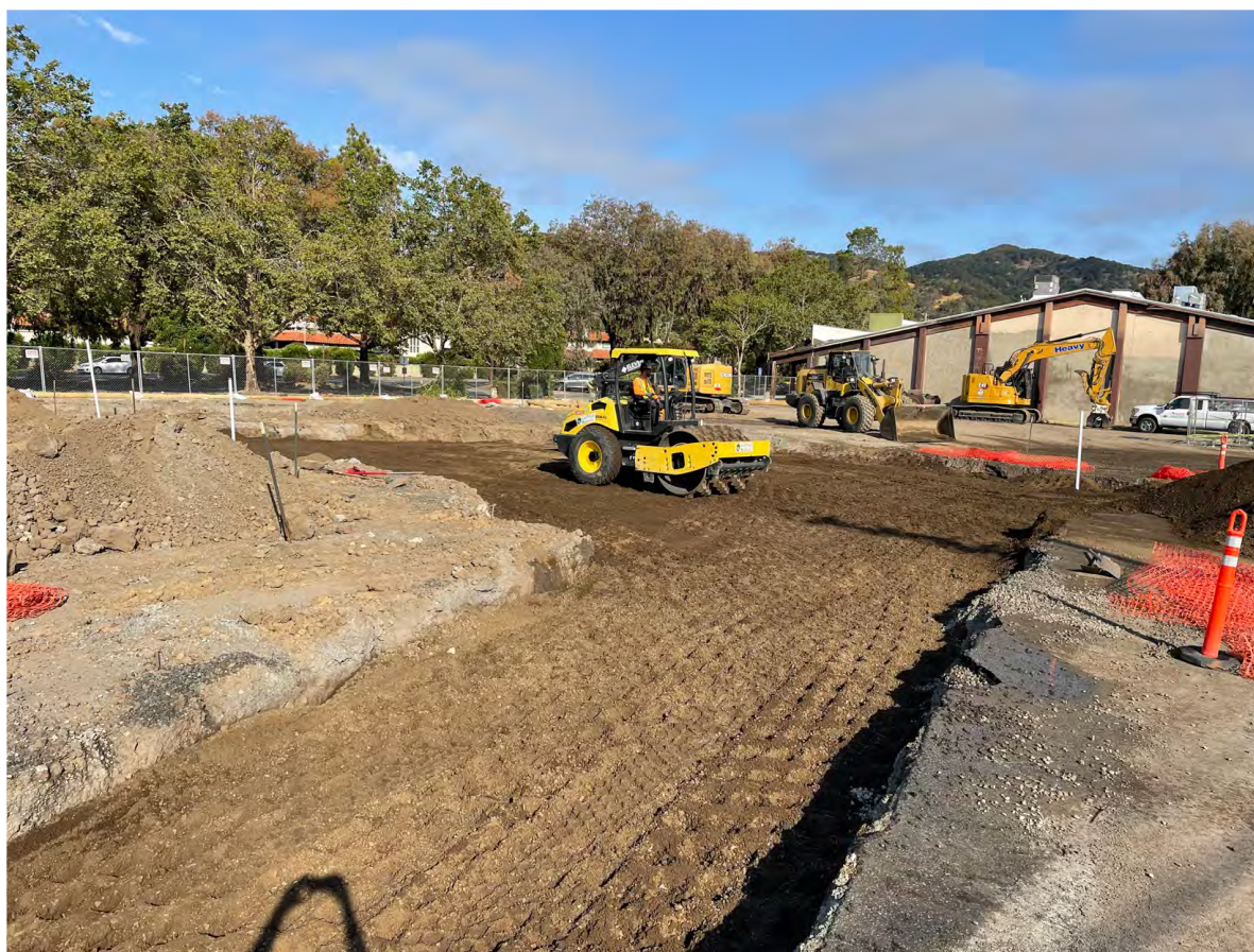
Photo showing excavation backfill at the former dry cleaner building location
