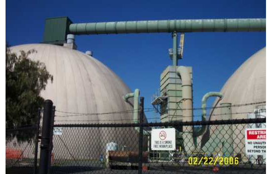
Coke is transferred via a fully enclosed system
