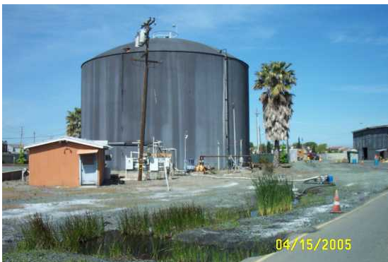
1,000,000-gallon tank used to store stormwater
