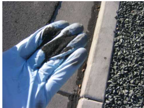
Close-up of coke found in curb
