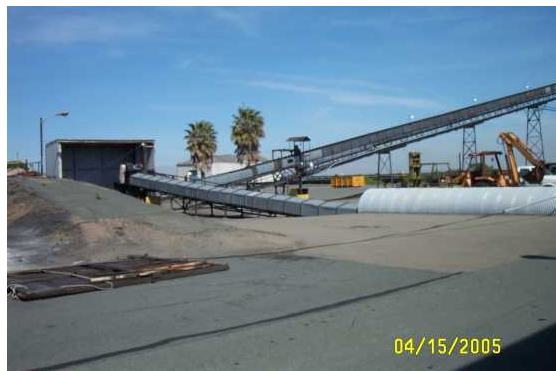
Second covered conveyor system transfers coke from stockyard area to ships
