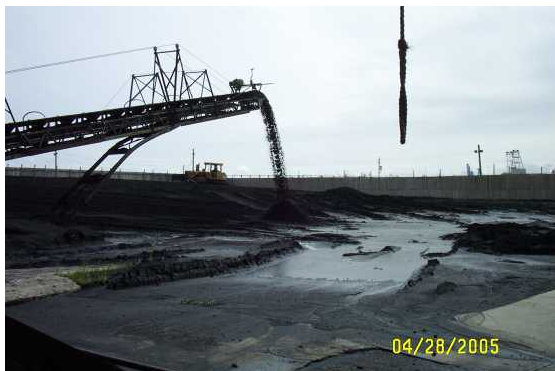
Coke is sprayed with oil for dust control before being deposited into the stockyard area
