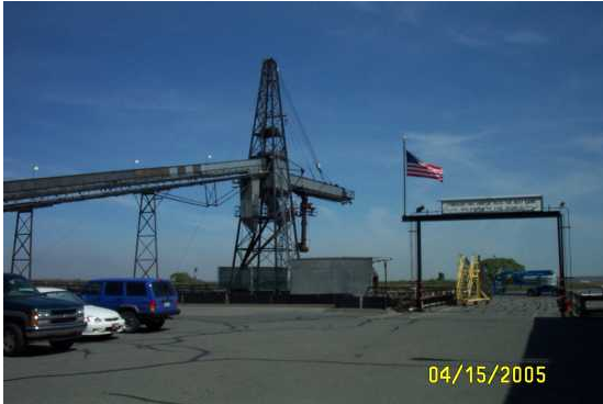
Covered conveyor leading to loading chute
