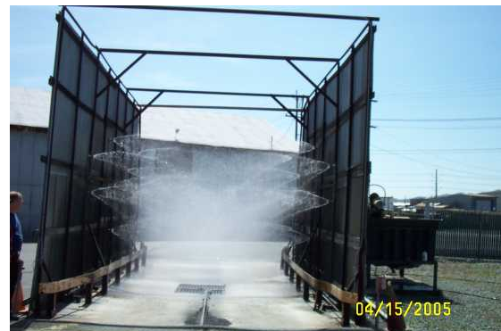
Wash station used to clean trucks before they leave the facility
