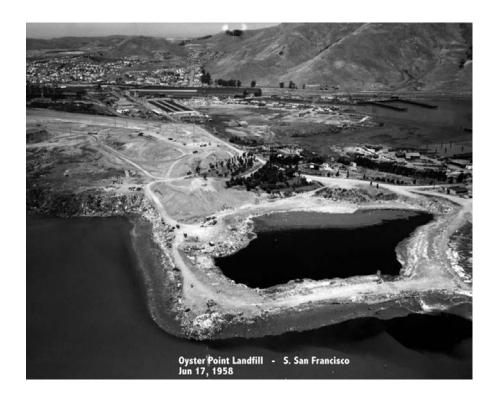
As late as the 1960's, Landfills were constructed into the Bay by placing earthen berms into the Bay and simply filling the center with waste.
