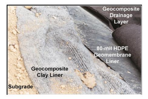
Present-day standards require engineered designs consisting of liners with multiple components. The above is for a sideslope, where yet another High Density Polyethyene (HDPE) layer will be put on top of what is shown here.
