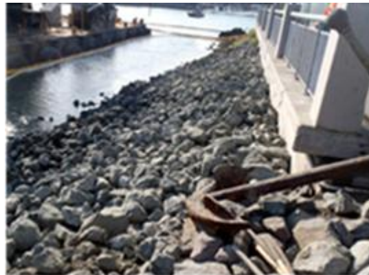
Photo 2e. Finished slope.
