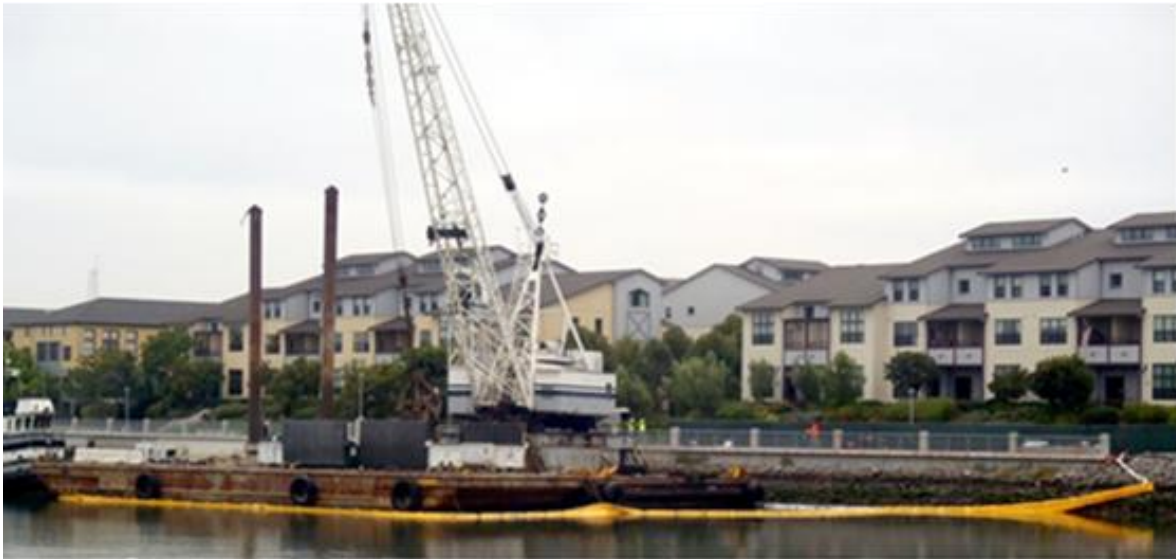
Photo 2a. Barge-rig-boom layout from the Alameda side of the Oakland Estuary.
