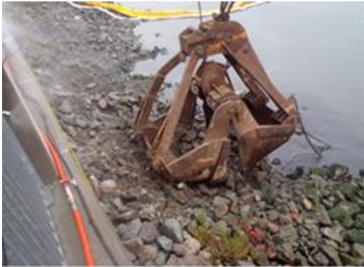
Photo 2b. Exposing impacted soil under the riprap.
