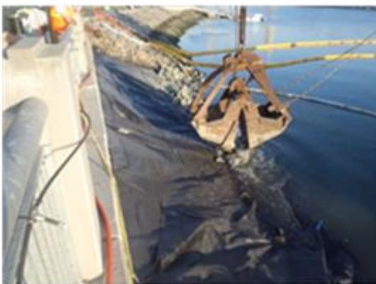
Photo 2d. Securing the new geomembrane.
