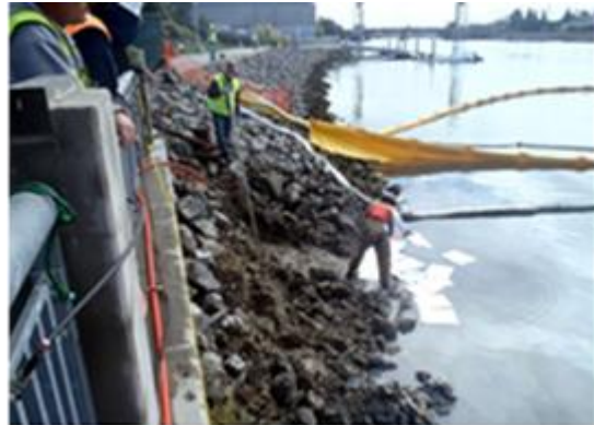
Photo 2c. Exposing the end of the existing geomembrane.
