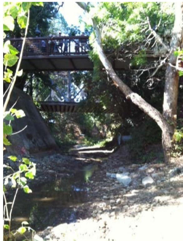
Photo 1b. Creek after barrier removal.
