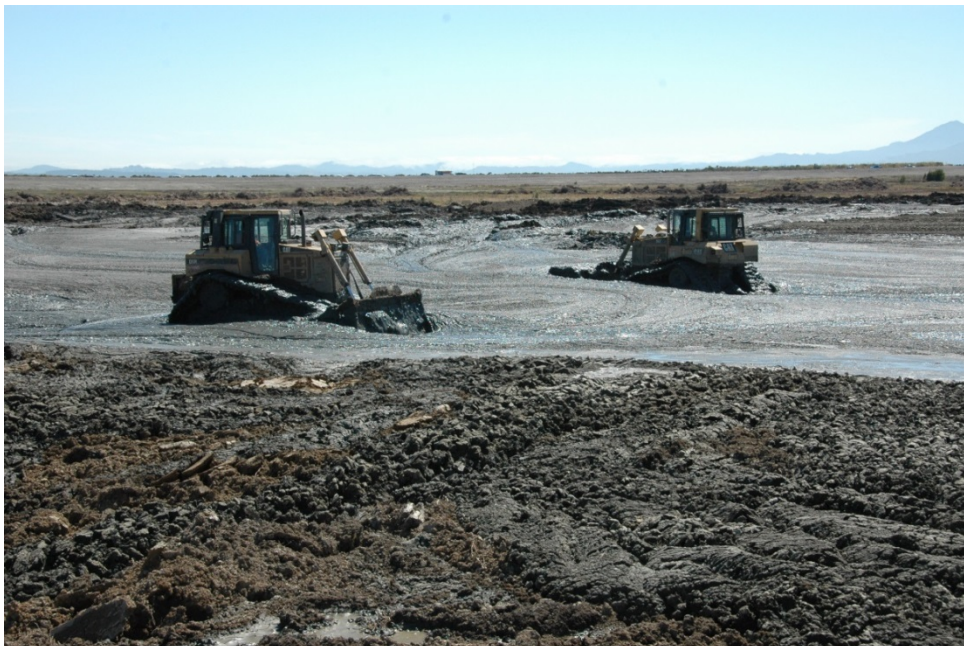
Photo 1d. Bulldozers spreading Mare Island dredged material at Cullinan Ranch.
