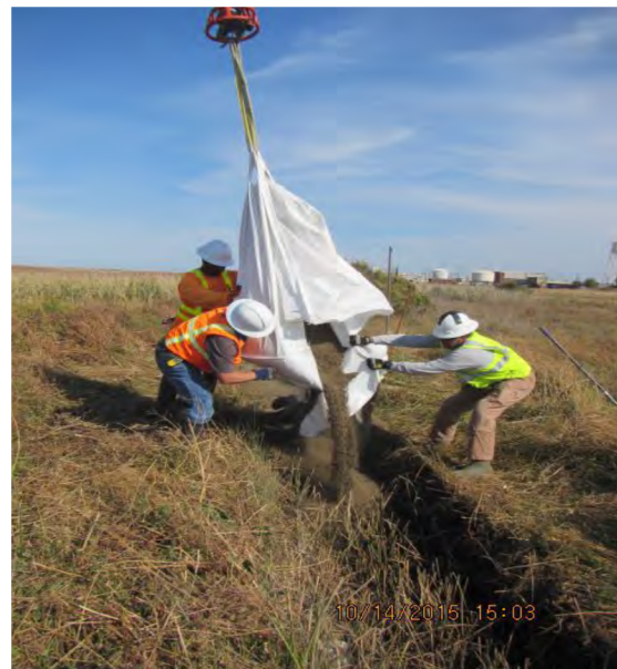
Figure 1c. Placing of the cap material.
