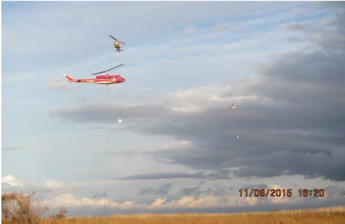
Figure 1a. Long-line helicopters delivering clay to the sloughs at MOTCO.
